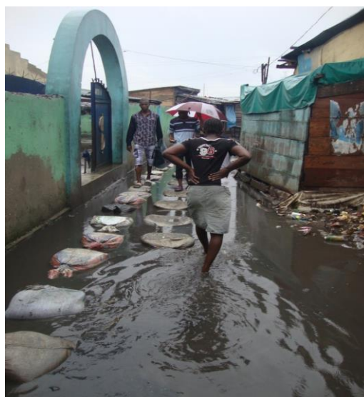
Figure 4. Filling with Sandbags in Ago-Egun neighborhood.
