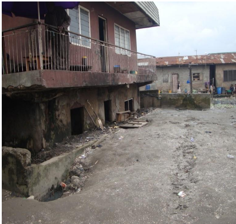
Figure 6. Construction over existing sunken house.
