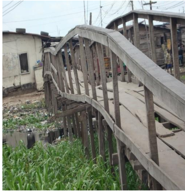
Figure 5. An example of a constructed communal wooden walkway.
