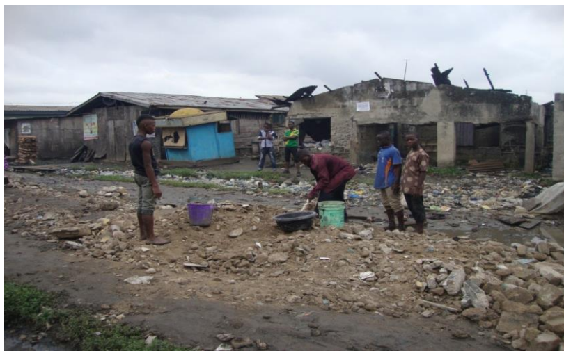
Figure 3. Filling with broken blocks at Isale-Iwaya neighborhood.
