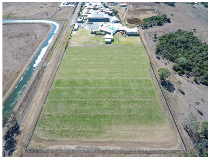
Figure 4. Aerial image of Bundaberg Christian College's oval.
