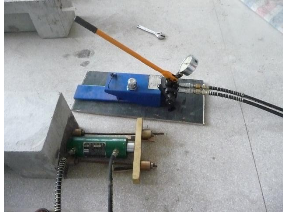
Figure 5. Tensioning of the external tendon.
