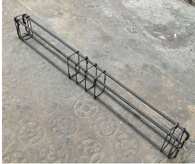
Figure 7. Beam reinforcement view.
