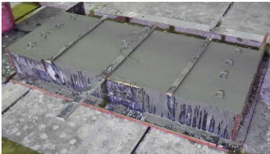
Figure 8. RC beam construction.
