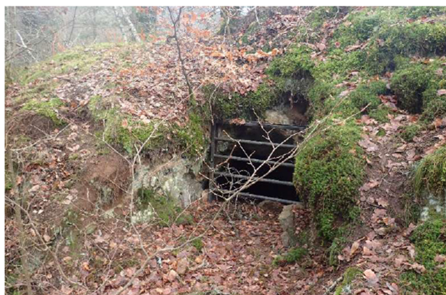
Figure 4. Entrance to galleries serving as a bat roost [8].
