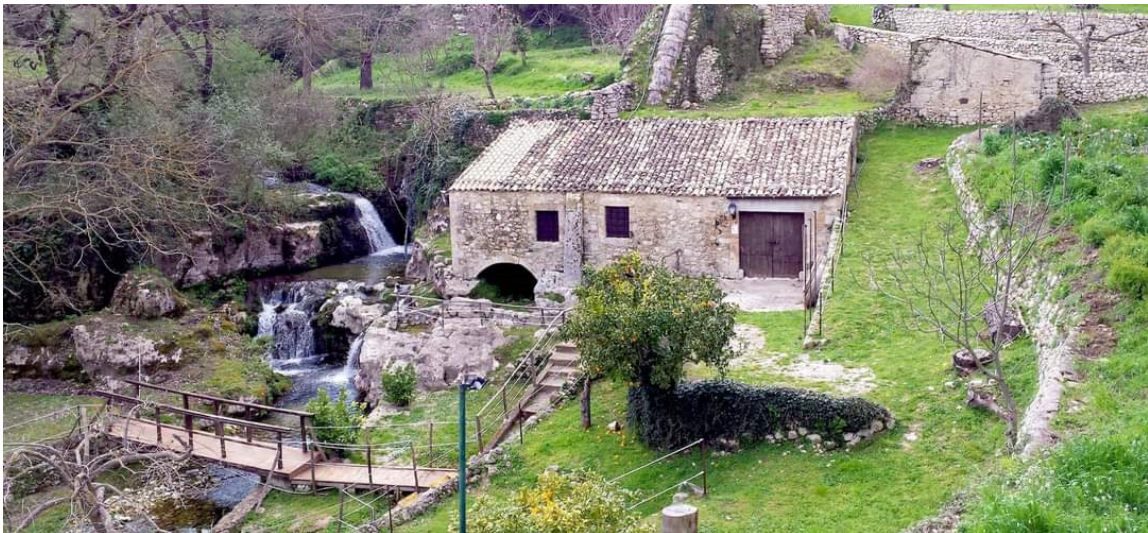
Figure 3. The water mill Santa Lucia as a site within the ecomuseum in the municipal territory of Palazzolo Acreide.
