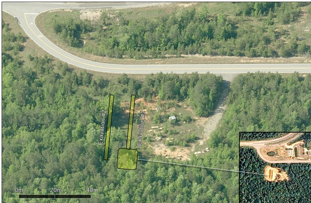
Figure 3. NGES aerial with approximate excavation locations [2].
