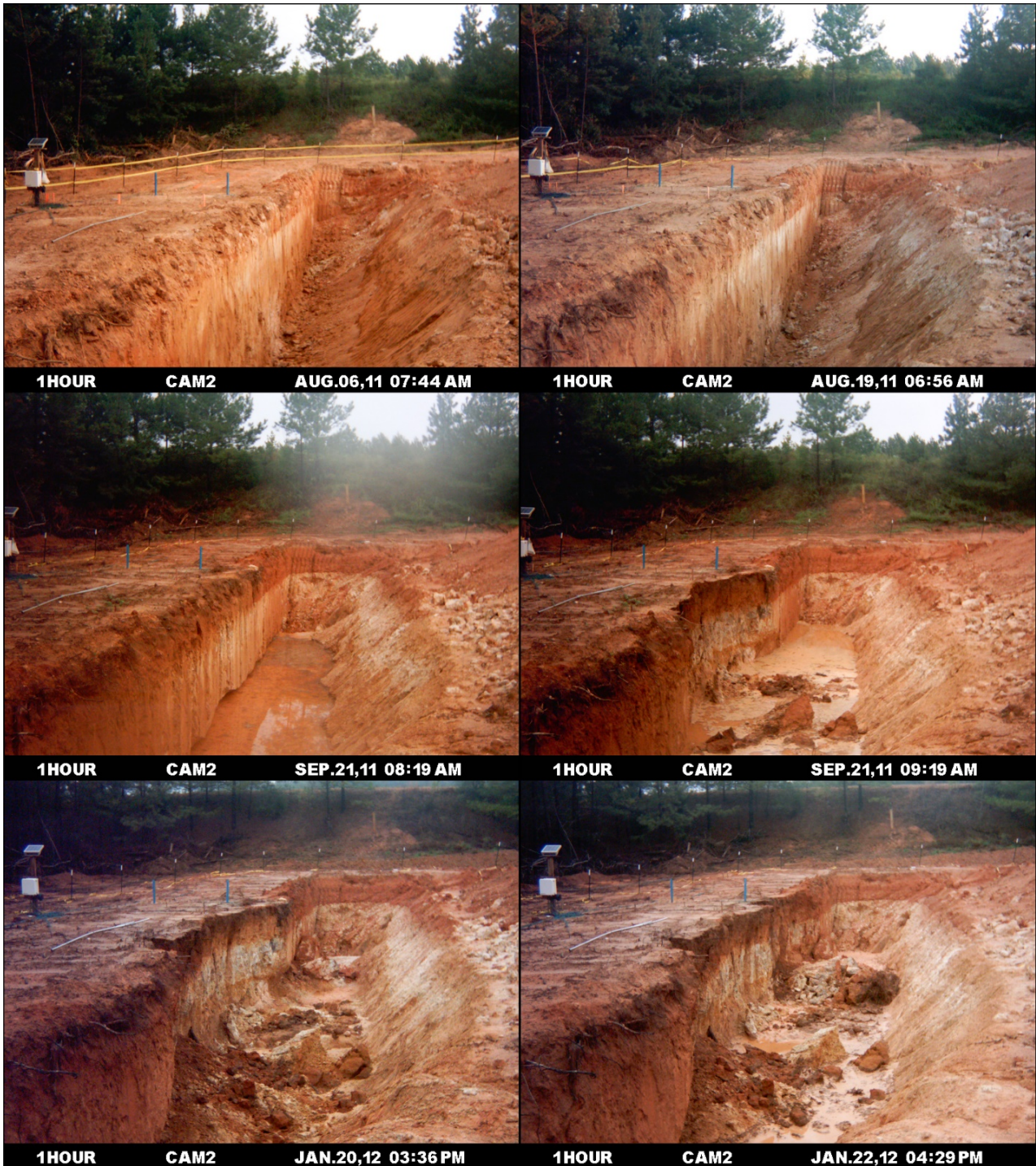
Figure 9. Excavation #2 time-lapse photos before and after failure.
