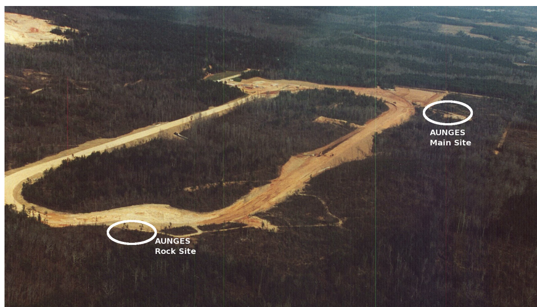
Figure 2. Early construction photo of the test track looking from the southwest (Photo courtesy of the National Center for Asphalt Technology).
