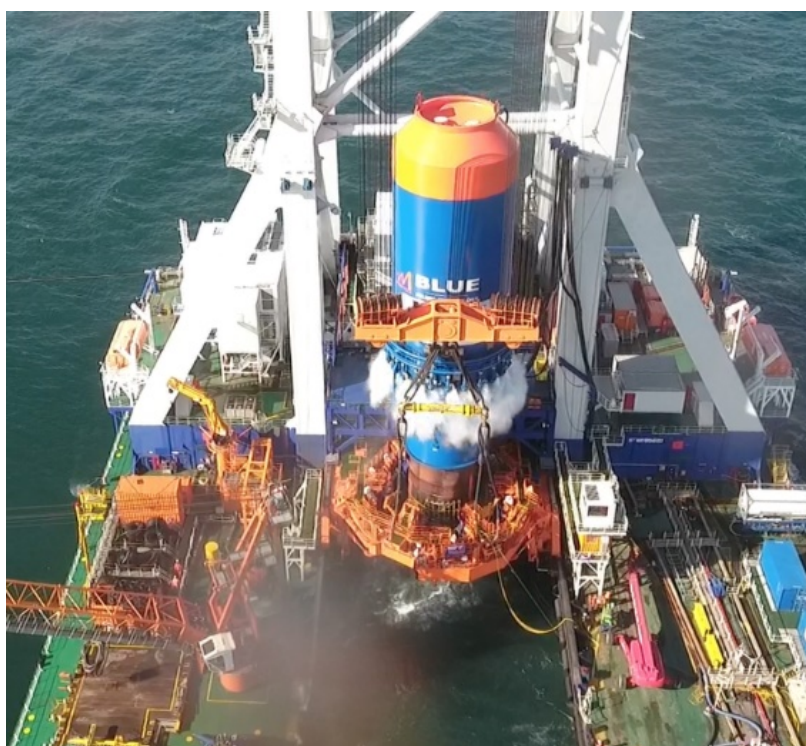
Figure 4. Offshore trial of BLUE 25M hammer (courtesy of Fistuca BV).
