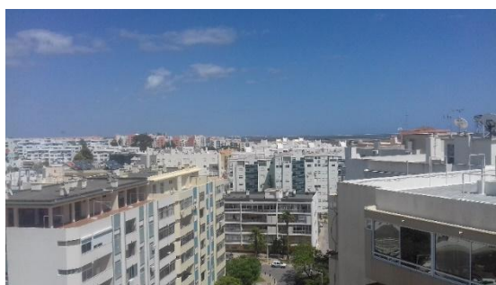
Figure 3. Flat rooftops in contiguous buildings in the city of Faro.
