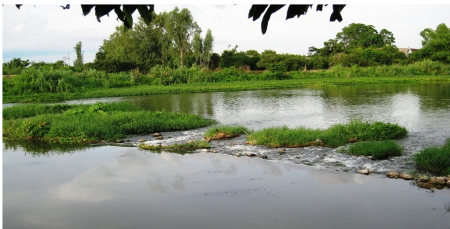
Figure 2. The muang fai Sop Rong headwork area.
