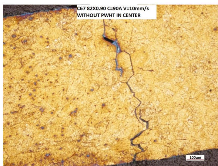
Figure 6. A crack was found in the melting zone area when the welding was performed without PWHT.
