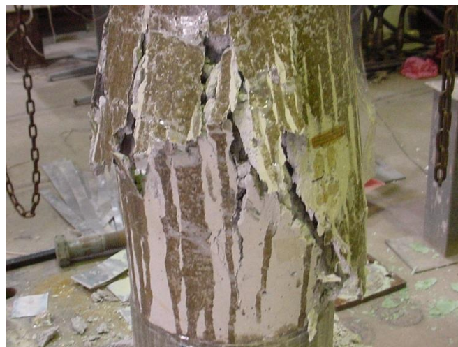
Figure 14. Spalling of un-corroded OPC concrete column at failure during structural test.
