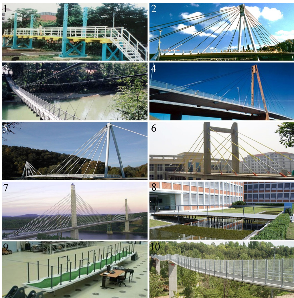
Figure 2. Existing CFRP cable structures.
