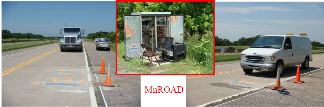
Figure 21. Installation of CNT/cement sensor in roads for testing monitoring capability.
