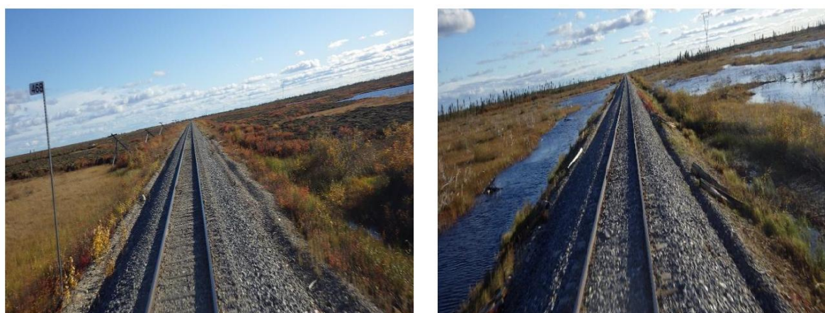
Figure 6. Photos of milepost 468 (left) and milepost 448 (right) showing no tree cover and ponded water close to embankment shoulders.
