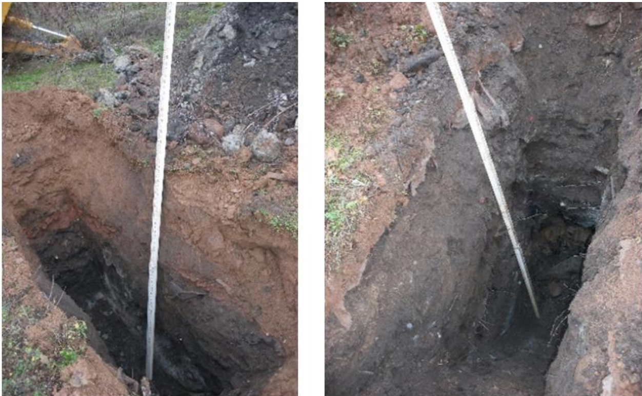
Figure 5. Soil test pits dug to ~4 m at Lion's Gate Park wetland restoration site showing non-heterogeneous unknown fill material depth layers.
