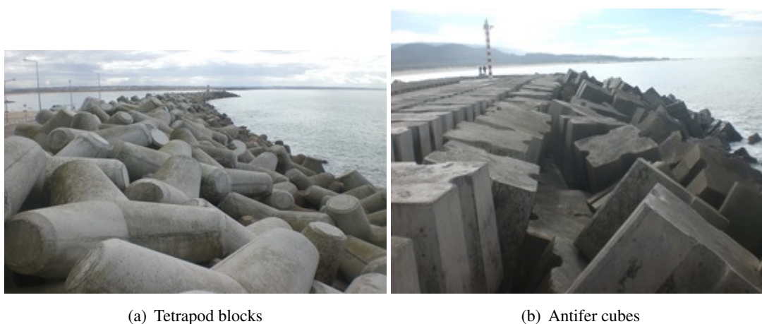
Figure 1. Rubble-mound breakwaters armour layers consisting on concrete blocks.
