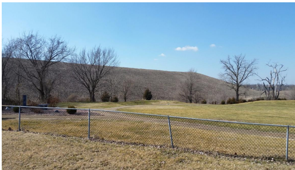
Figure 2. Image showing quarry stone covering the surface of the remediated Bonne Terre chat pile. Photograph taken by author on February 13, 2016.
