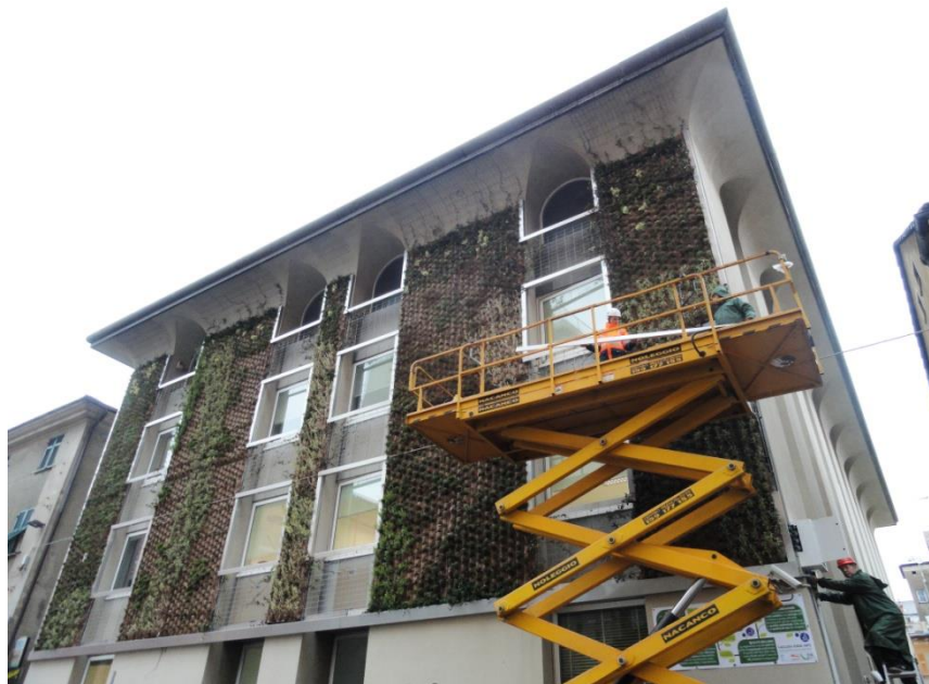
Figure 2. The green facade during construction.
