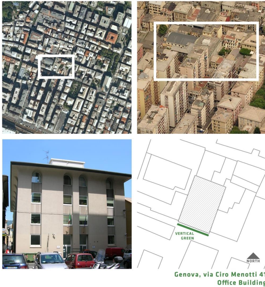
Figure 1. INPS office building location in a dense urban area in Genoa, Italy.
