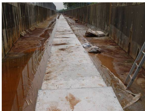
Figure 5. Construction of BioIronTech biofilter in the drain of polluted stormwater.
