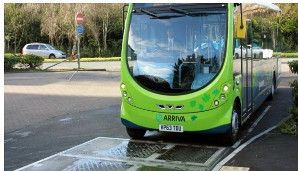
Figure 12. Milton keynes inductive charging system with pads [38].
