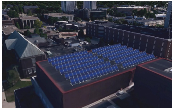
Figure 2. 3D rendering of Center for Performing Arts rooftop PV system.
