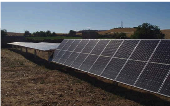
Figure 3. PV panels structures with hand-driven hor. axis regulation. Source [19].
