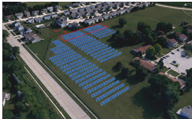
Figure 4. 3D rendering of Center for Renewable Energy ground mounted PV system (phase one system size outlined in red color).
