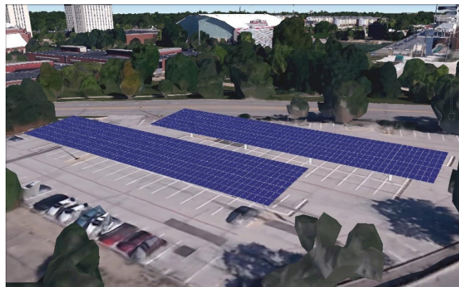
Figure 2. 3D rendering of Kingsley (G53) parking lot PV canopy system.
